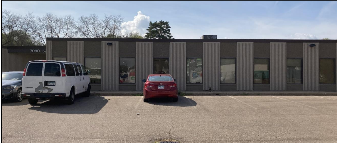
East side of building facing parking lot
