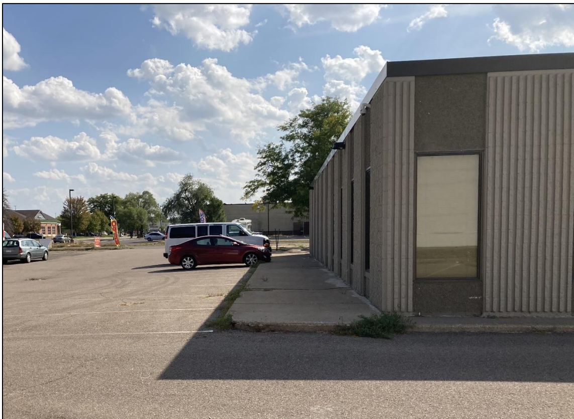
Looking south at parking lot
