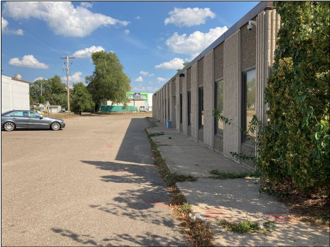
North side of property
